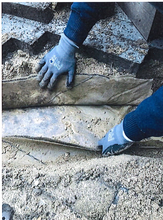
Foto 21: Membran under fibertex.
